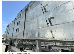
With trapezoidal bending for aggregate bin covers a high strength can be reached. In SEMIX's aggregate storage hoppers, extra reinforcement steels are welded to the empty spaces in the trapezoid. Thanks to this method, aggregate storage bins can serve long years.
